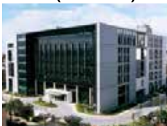
Taoyuan Technology Center (Green Building)
